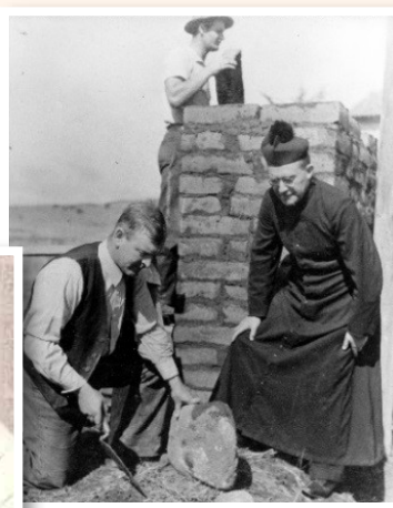
Harry Downie and Fr. Michael O'Connell doing restoration work in 1939. John Yementes is laying adobe bricks.
