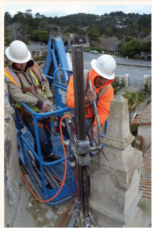
Drilling cores for steel rods
