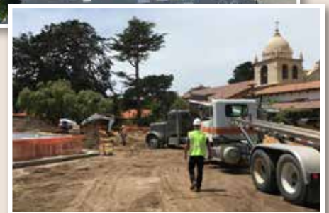
The 2016 Quadrangle Courtyard renovation was the first major project of Phase II.
