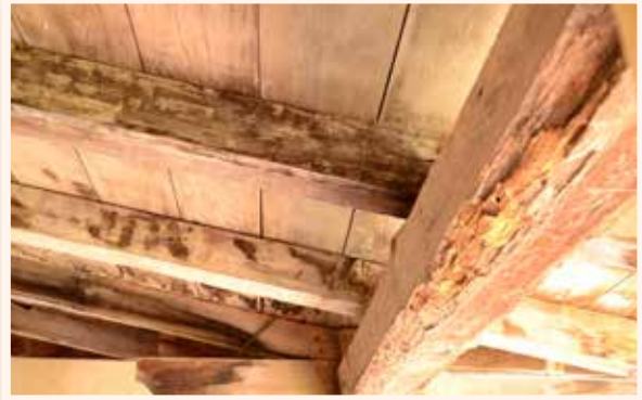
Deteriorating wooden beams in Convento Museum
