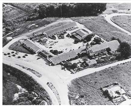
1946 Mission restoration in progress
