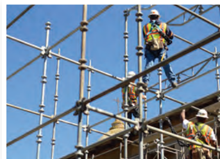
Workers assembling scaffolding. Photo by Doug Mueller
