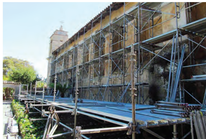
Scaffolding going up around the Basilica. Photo by Blach Construction
